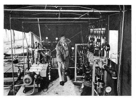
RUSS MAXWELL (2165) inspects pumping system and valves for air, fuel and water for Deep Steam. This equipment, mounted on a skid, will be moved to Long Beach site along with another module which contains the control equipment.
